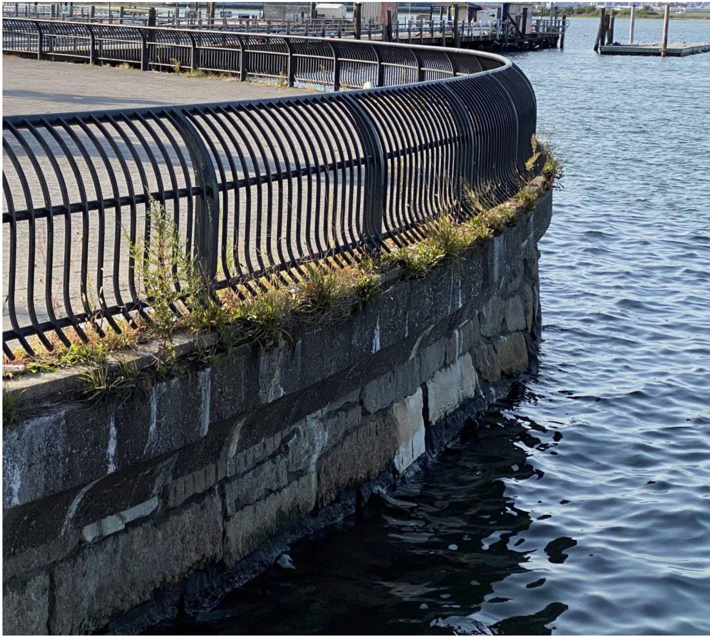
Deteriorating Bulkhead
